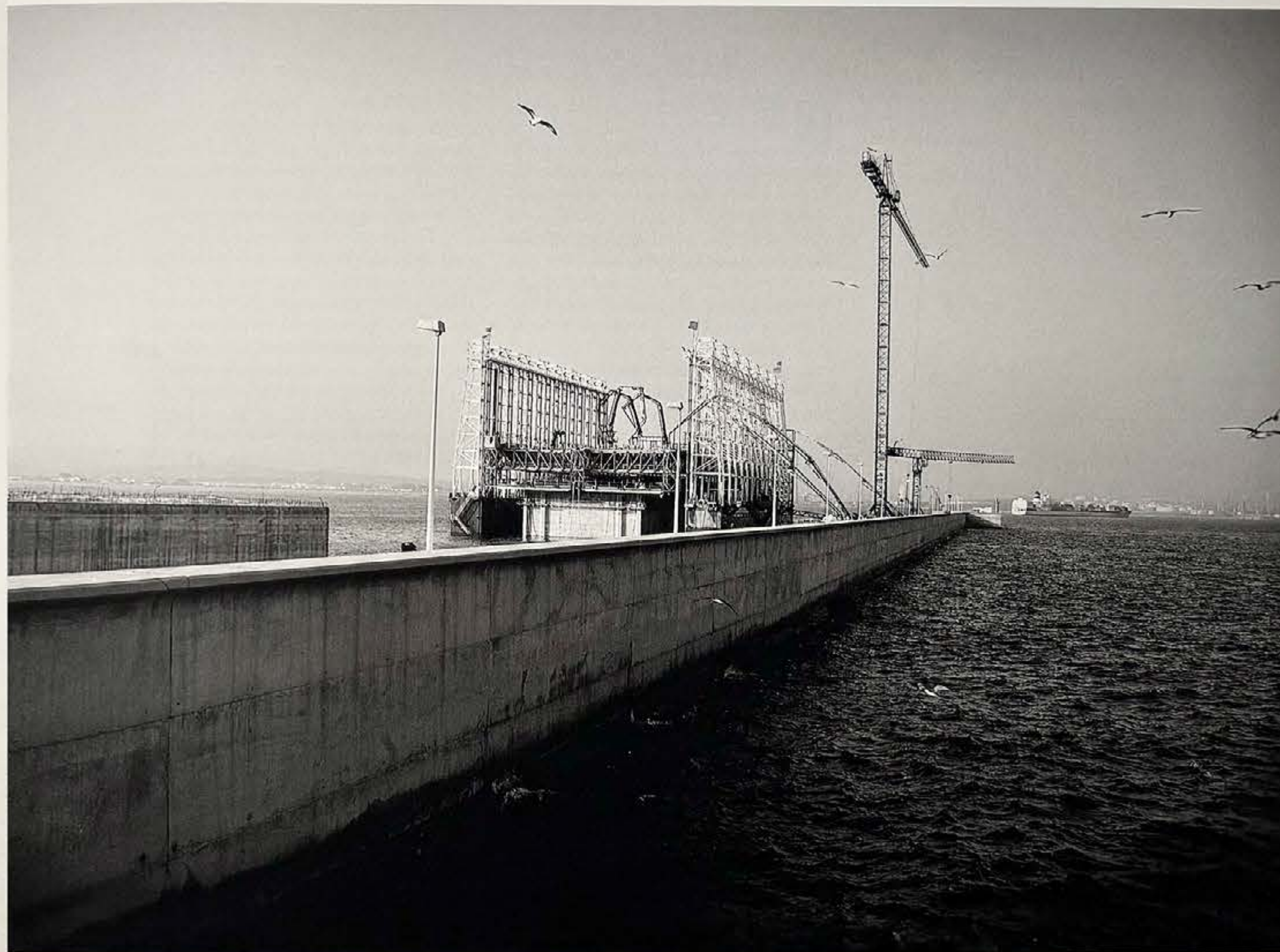
A new detached breakwater is currently being built to protect the new Isla Verde Exterior quay. The photograph shows the Kugira floating dock, which manufactures Europe's biggest caissons, measuring 67 x 24 x 29 metres, using this method. 2007. (Photo: Víctor Román)
